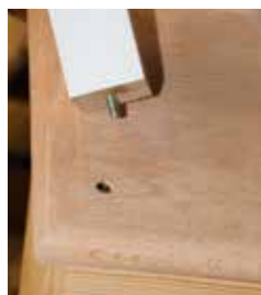
Treads are drilled for balusters, and inserts are installed.
