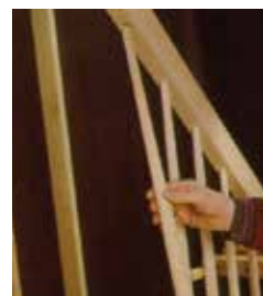
Rake rails on stair are drilled for easy baluster insertion, up into rail and down into tread.
