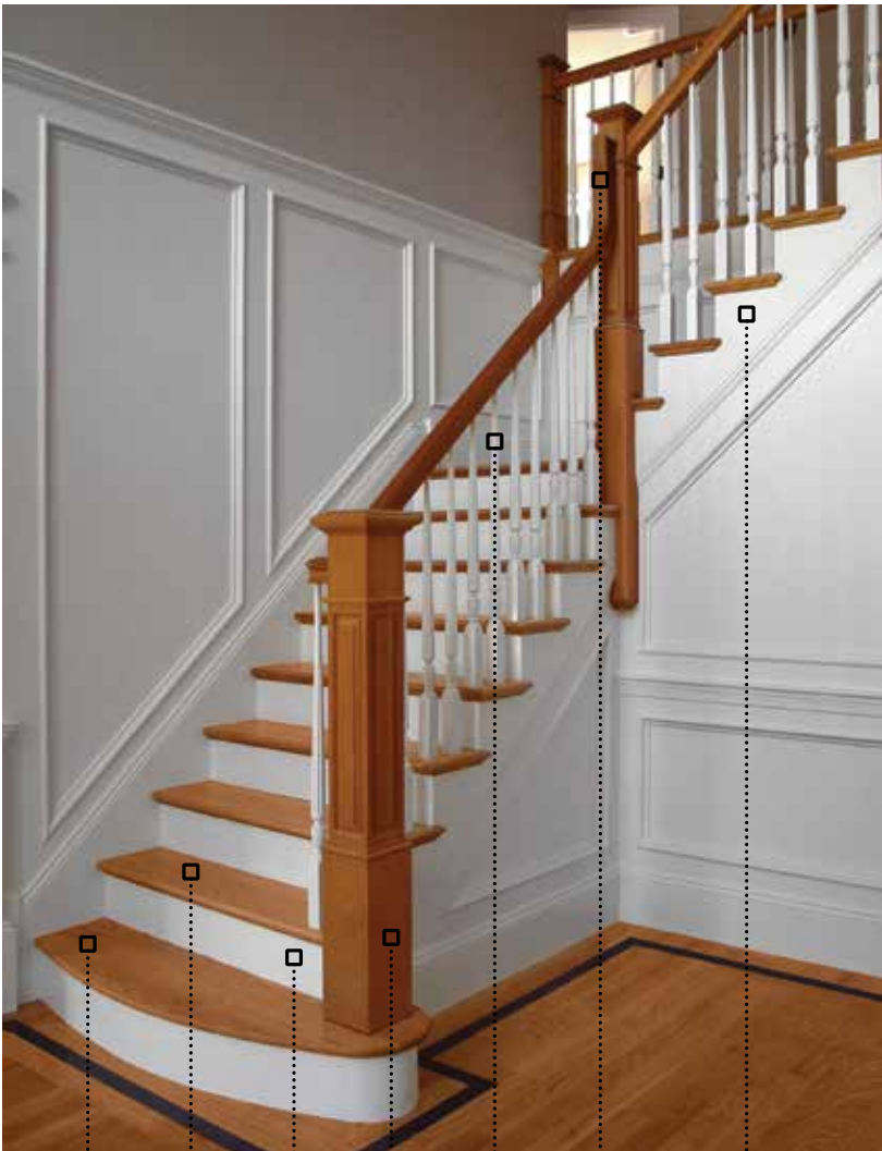
Starting Step Tread Riser Box Newel Wood Baluster Gooseneck Stringer
