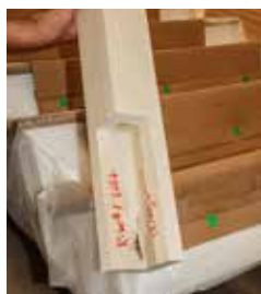
Post is notched for exact location and height.
